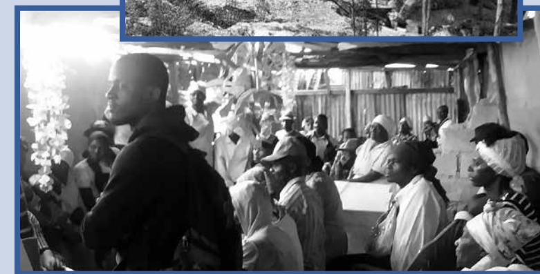
Left to right: Top and middle photo: Beginning foundation of new church/school/clinic at Soliette in Haiti. The new building is being built around the original building. Bottom photo: People of Soliette wait to see the doctor inside the old Our Lady of Grace Church and clinic.
